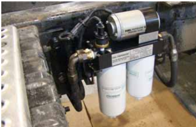
This installation on a short nose "Day Cab" is on the driver's side, behind the battery box.
